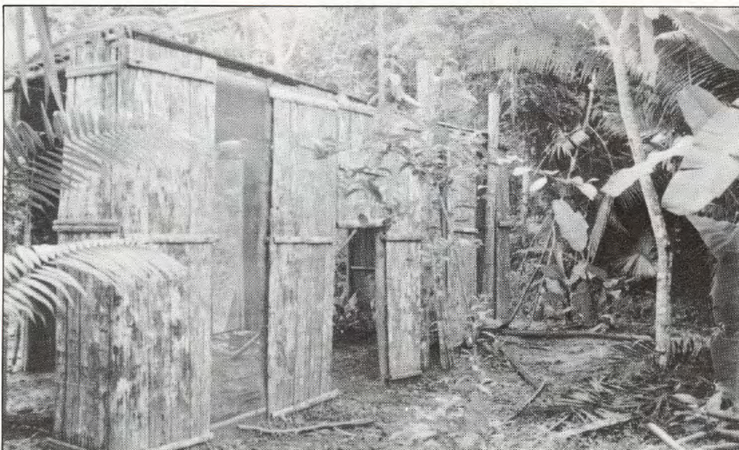
Macaw aviaries under construction in the Tambo Yarapo reserve
