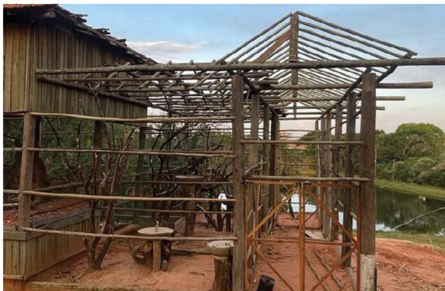
WPT-funded aviary under construction
